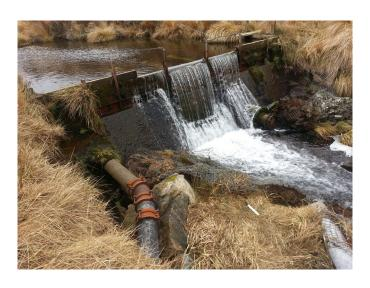
Photo above shows front wall of weir. You can just see floating below the calm water three white pipes, these are the filters.
